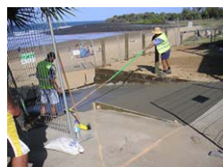
Left: pouring the concrete ramp
