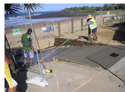
Above: Building of retaining wall Left: pouring the concrete ramp
